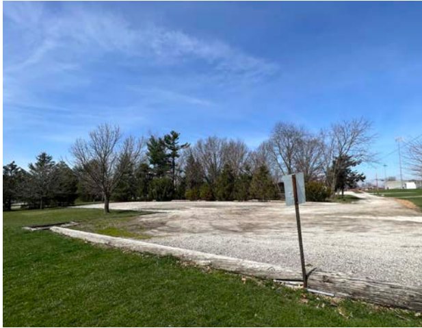
Northeast parking lot, entrance from Main St.
